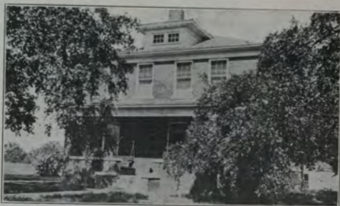
SUPERINTENDANT'S HOUSE, STATE FISH HATCHERY, ARMSTRONG, OKLAHOMA
