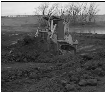
A bulldozer is the most cost-efficient tool when excavating a pond. The average rates for a bulldozer operator is $85 an hour or $1.50 per cubic yard removed.
