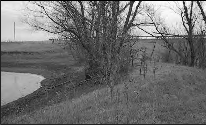
Having trees on your pond dam can be a serious problem. It's not a bad idea to remove them when renovating your pond, but be careful. Water likes to follow the channels of rotted tree roots through the dam, causing the backside of the dam to slide.
