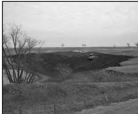
A bulldozer is the most cost-efficient tool when excavating a pond. The average rates for a bulldozer operator is $85 an hour or $1.50 per cubic yard removed.
