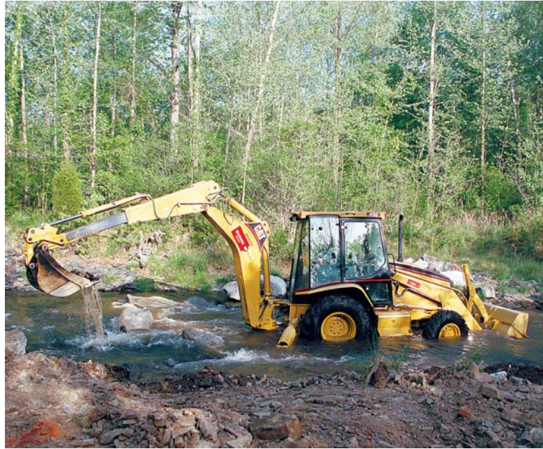
Heavy equipment was used to create ideal fish habitat and angling conditions.
