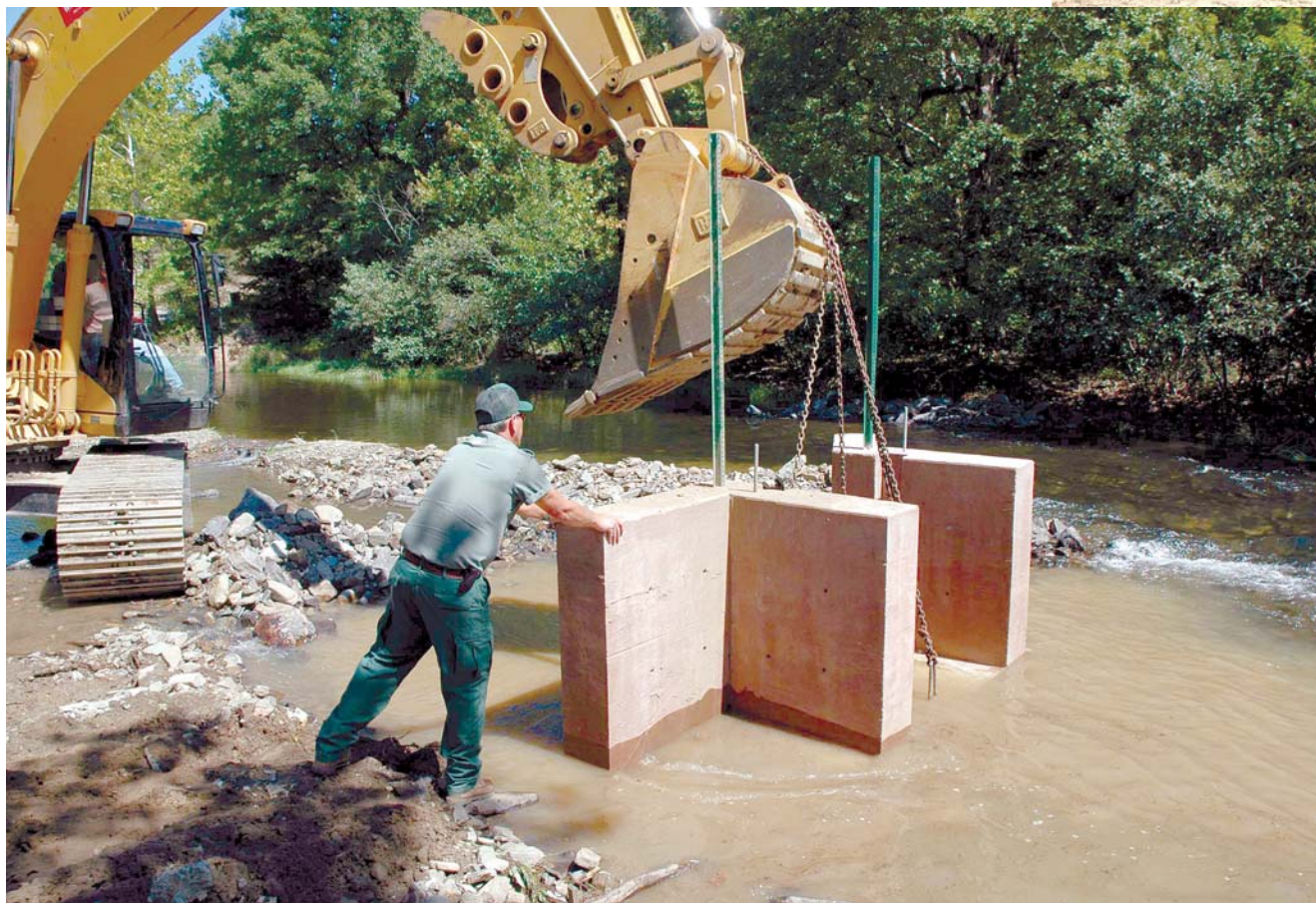
A large structure was put in the streambed to divert some of the water flow into the new stream.
