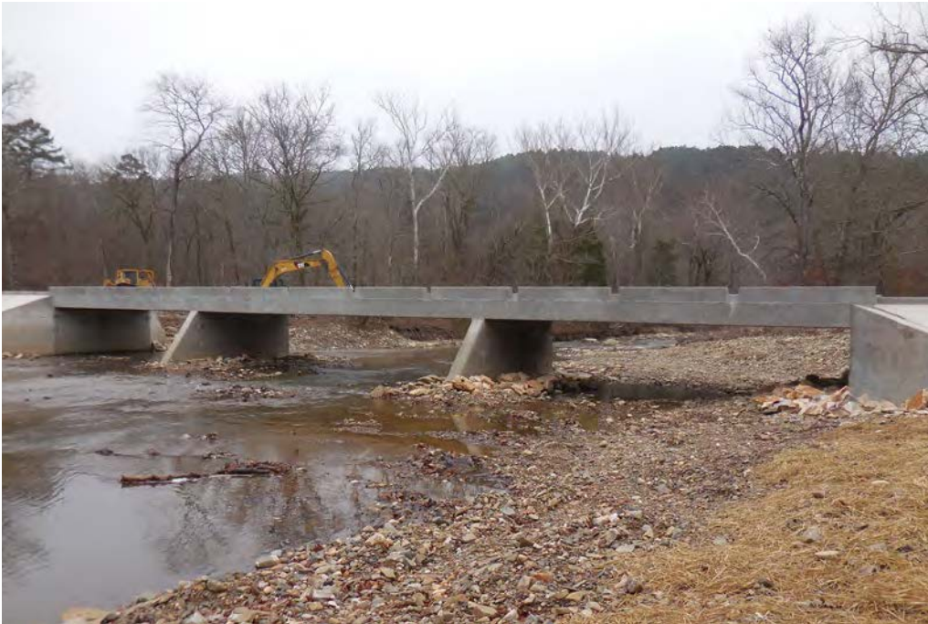
The U.S. Forest Service renovated a 1950s-era crossing on Cedar Creek to allow for a more free-flowing river and fish and freshwater mussel communities. Photo by Joe Vacirca/USFS.
