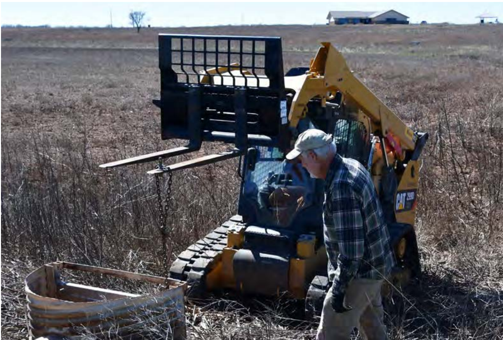
Biologists replaced flashboard risers at Hackberry Flat Wildlife Management Area. Photo by Cheyenne Gonzales/ODWC.
