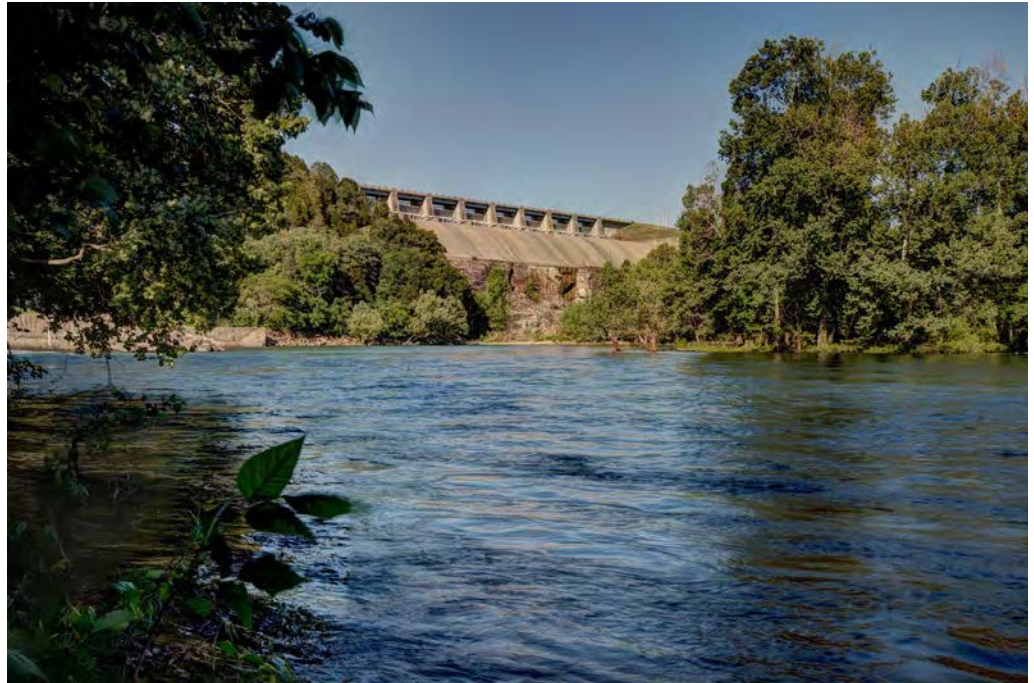
Tenkiller Ferry Dam at Tenkiller Lake in Sequoyah County, Oklahoma. Photo by ODWC.
