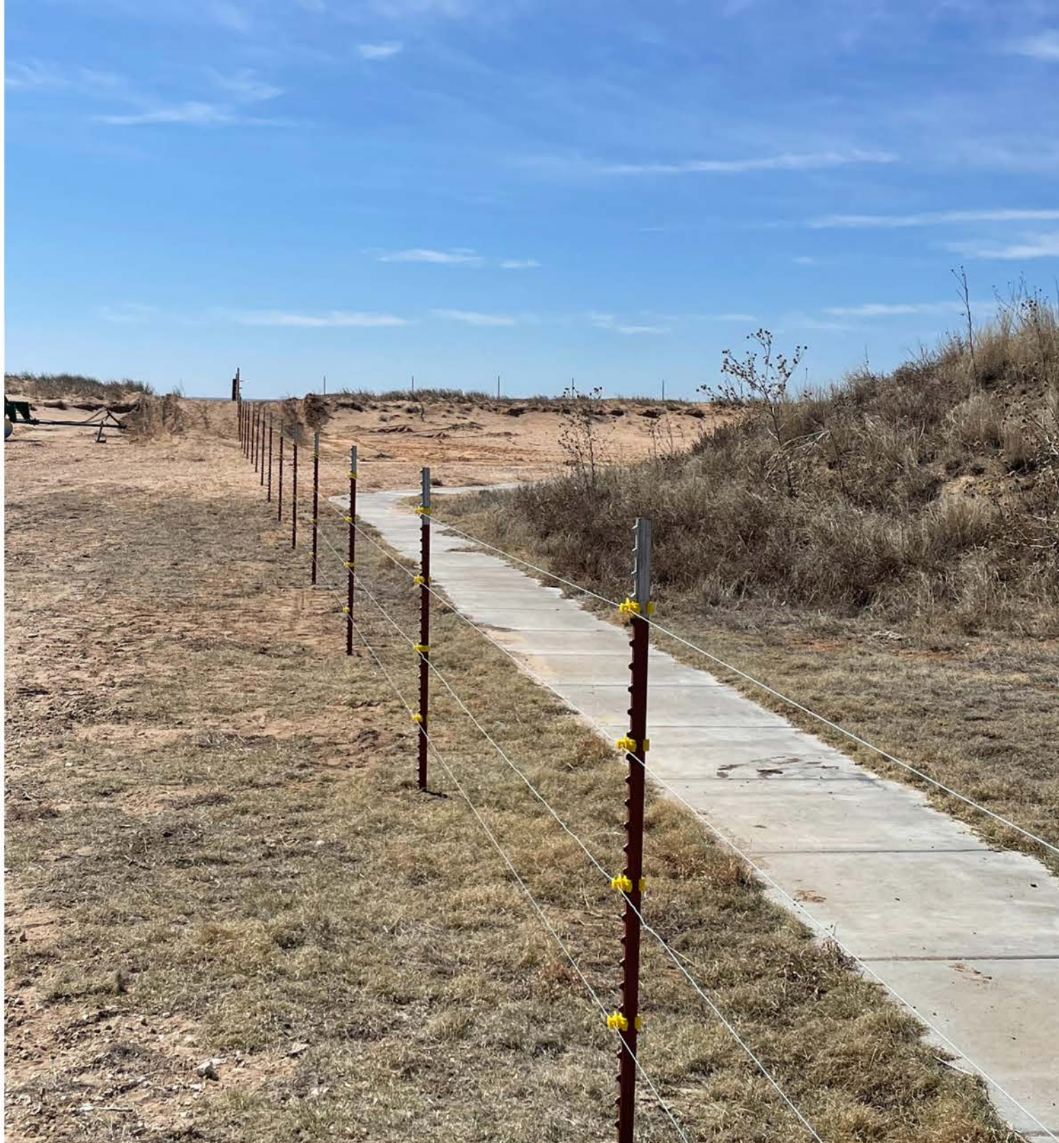
The new Beaver hotwire fence will keep out any wandering livestock.
