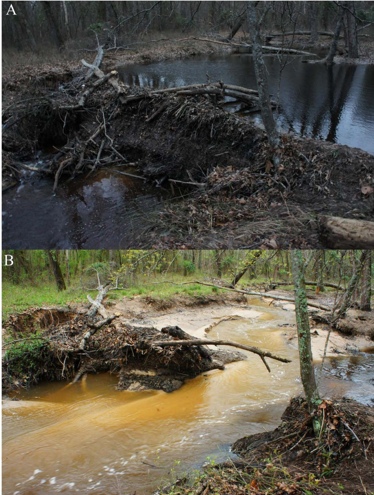
Figure 6. (A) A secondary dam built by TNC below both the current Boehler Lake dam and the original dam (4 February 2012). (B) A breach in the dam following a large storm (taken on 20 March 2012, the day after the breach).
