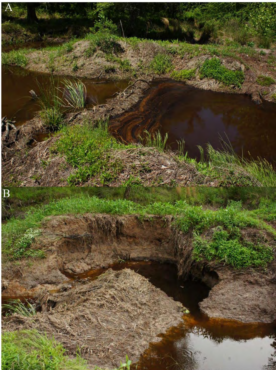
Figure 10. (A) A previous partial repair of the original dam at Boehler Lake (11 May 2013). (B) The original dam following a storm (taken on 23 May 2013, the day after the breach). The storm cut out the bank around the dam.
